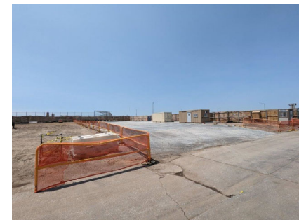
Site of trailer and future parking lot
