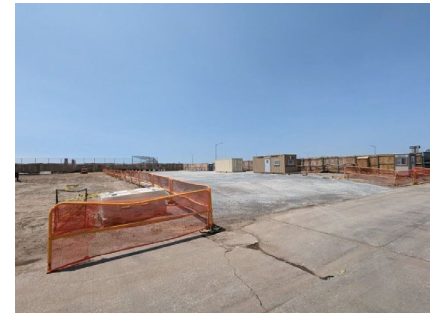
Site of trailer and future parking lot
